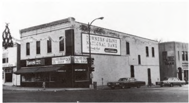
Southwest corner of Main and Curtiss Street — Late 1968
