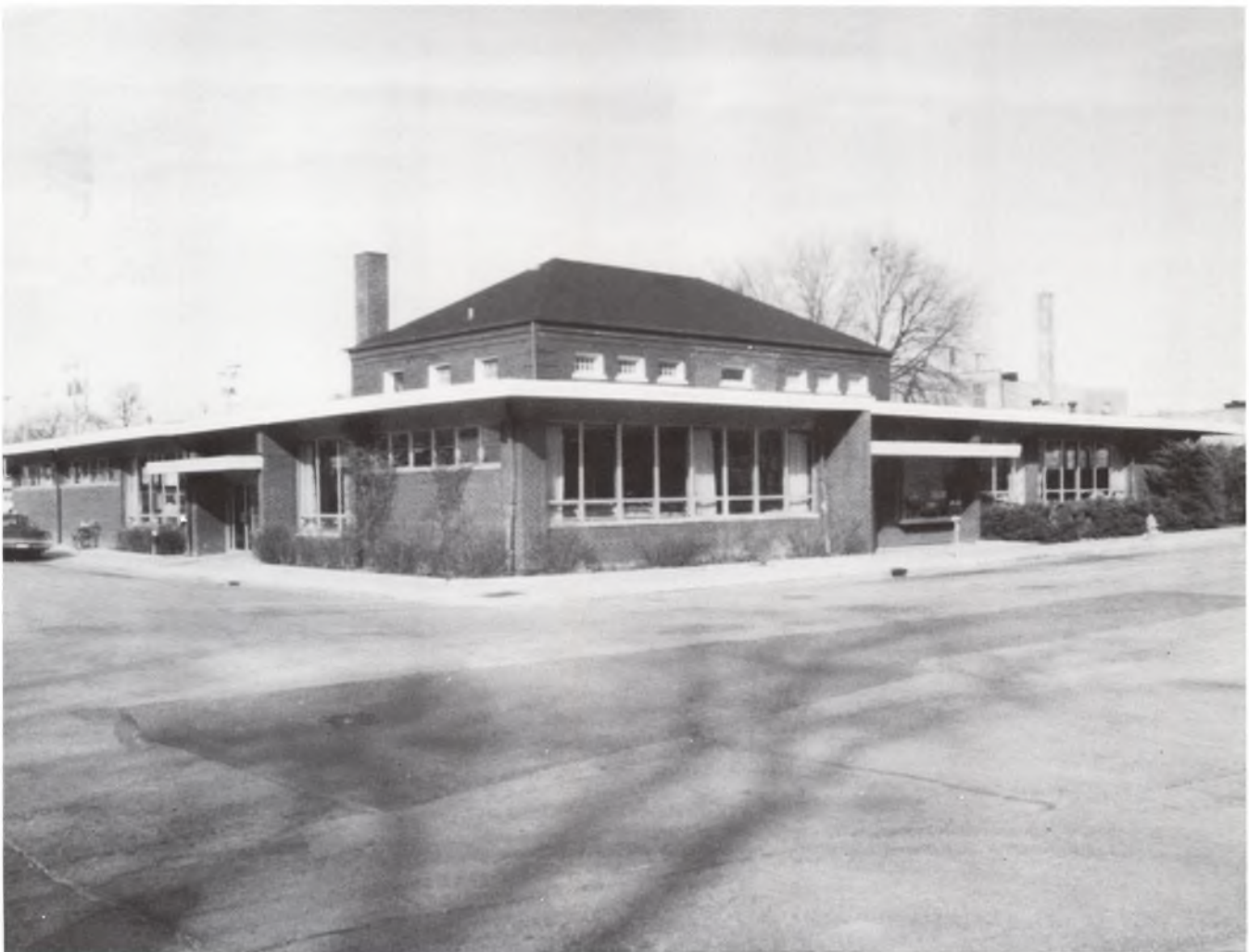
"Wrap-around" Library Building. Designed by George Steckmesser, Architect (photo by Robert Dunham)
