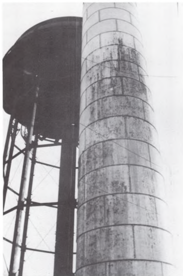
Old and new water towers side by side — old tower erected in 1894, new tower erected in 1938
