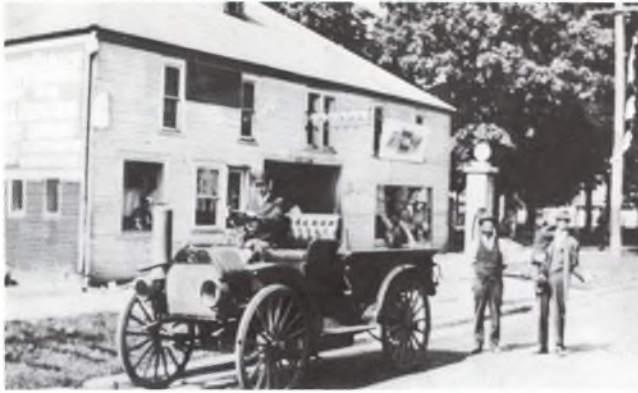
Old Crescy Auditorium, Grove and Main Streets
