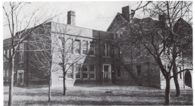
Washington School and addition
