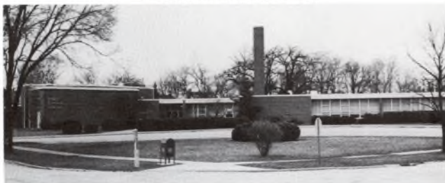
Stuart L. Johnson, Principal Pierce Downer Elementary School
