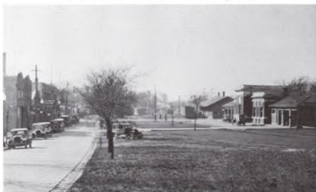
Both depots looking West at Main Street crossing
