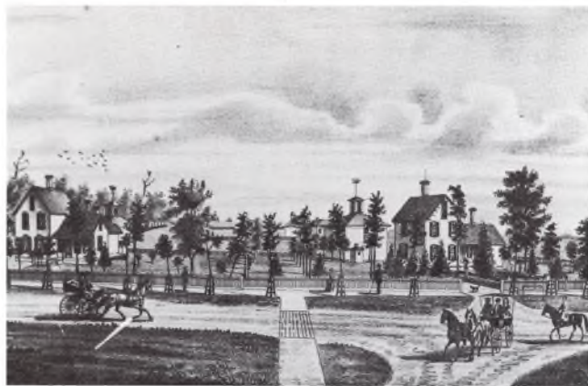
J. Warren Roger's house on the left and T.S. Roger's house on the right.
