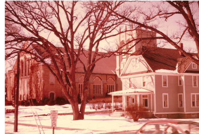
The former parsonage was located east of the sanctuary prior to being sold and moved in 1967 to make room for the building of the education wing and chapel.
